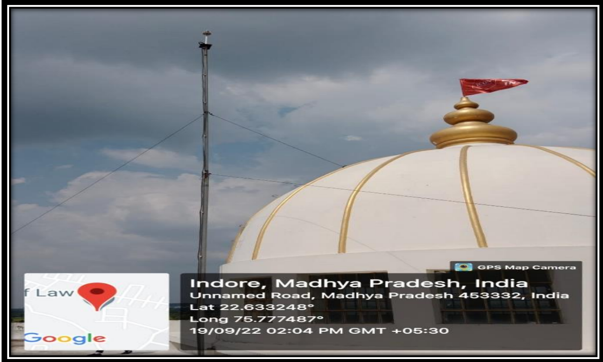
Installed Lightening Conductor in IIL Buildings
