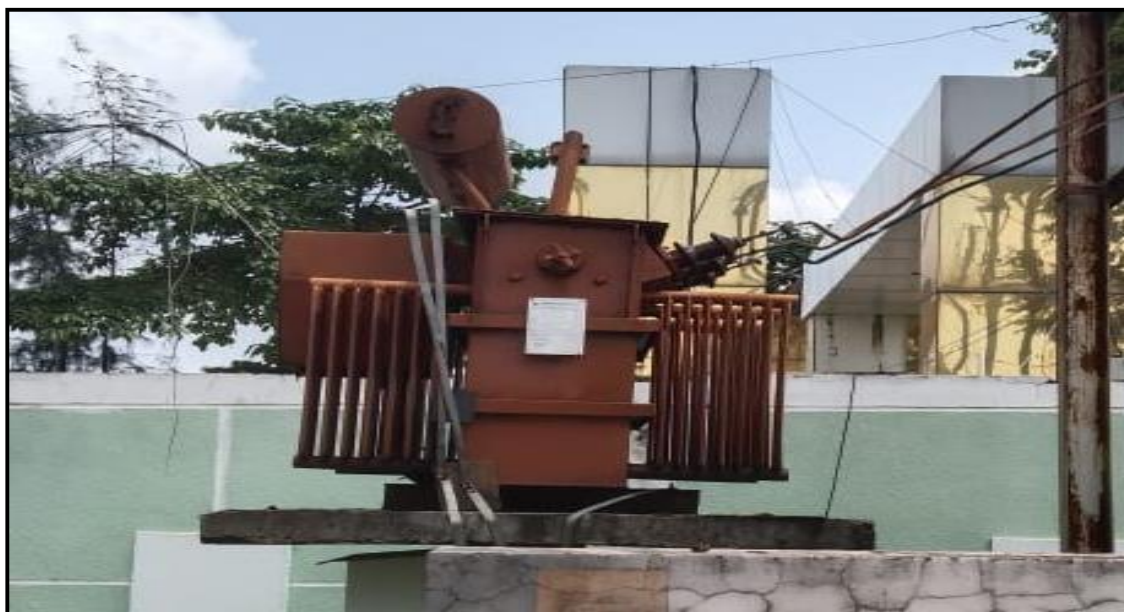
Figure 2.1:-315 kVA Transformer
